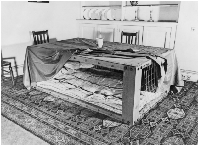
A Morrison shelter in a dining room, 1941
